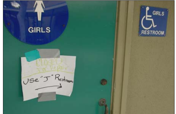
Girls Restroom in Building D
