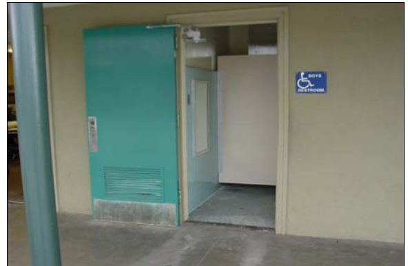
Boys Restroom in Building D
