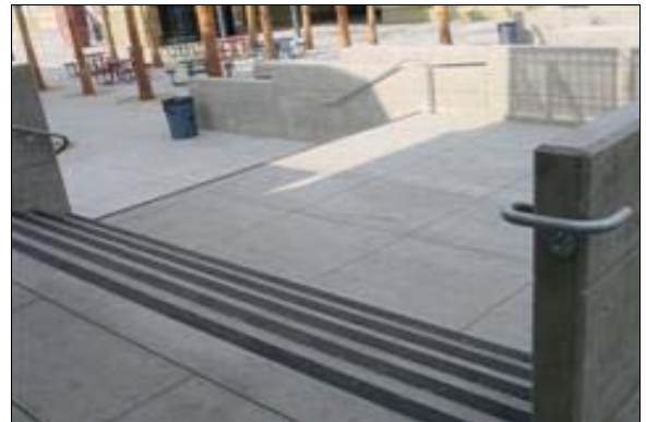
Stairs at Building 3
