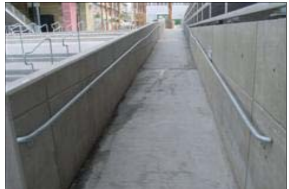
Ramp from Lucas Avenue
