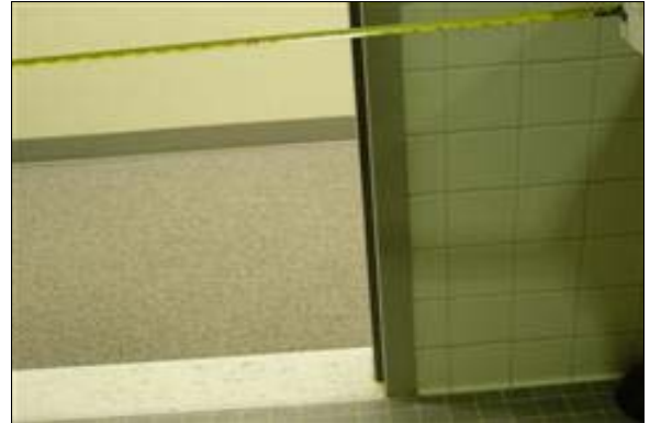
Unisex Staff Restroom in Office
