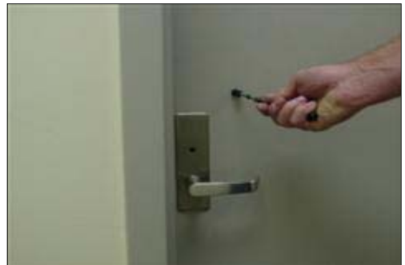
Unisex Staff Restroom in Office
