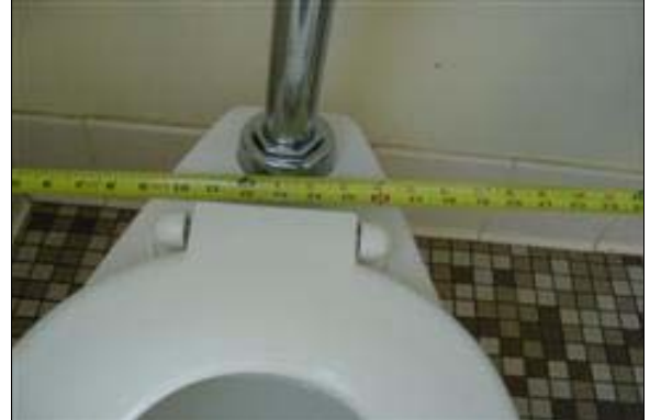
Unisex Restroom in Room 14
