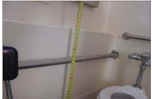
Unisex Restroom in Room 14
