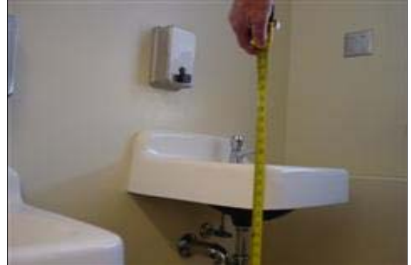
Unisex Restroom in Room 14
