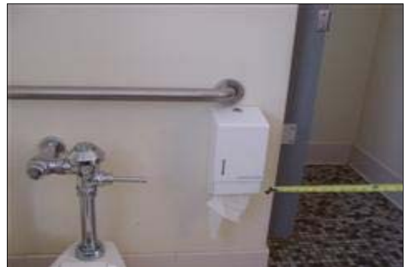
Unisex Restroom in Room 14
