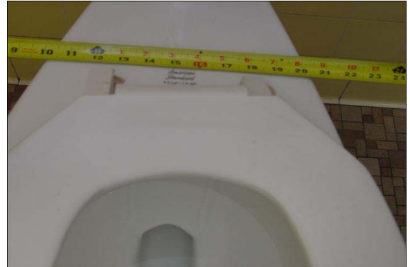
Boys Restroom Building A
