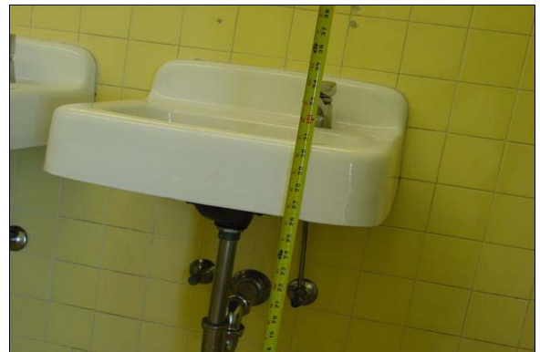
Boys Restroom Building A
