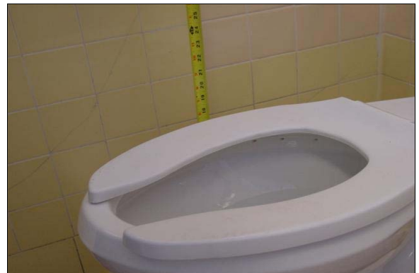
Boys Restroom Building A
