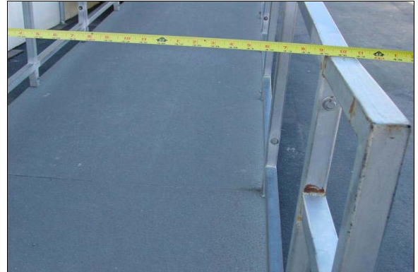
Ramp to Rooms 37 and 38
