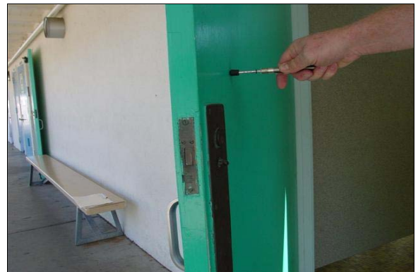
Girls Restroom Building A
