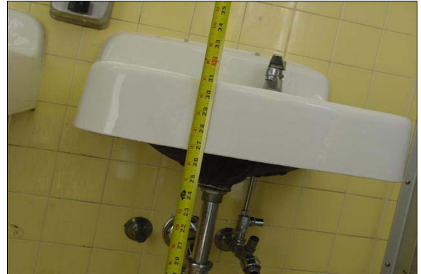
Girls Restroom Building A
