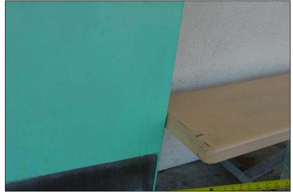
Boys Restroom Building A
