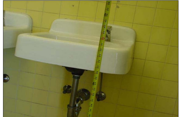
Boys Restroom Building A
