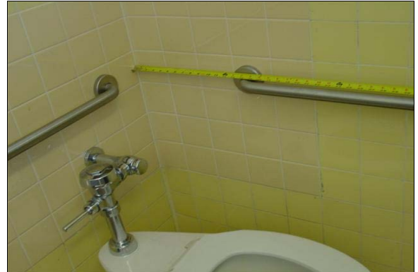
Girls Restroom Building A
