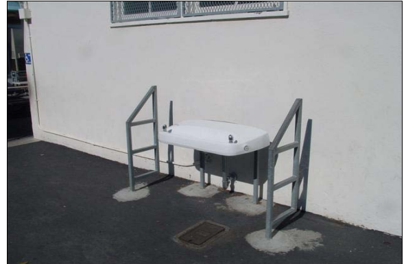
Drinking Fountain Near Girls Restroom at Building A
