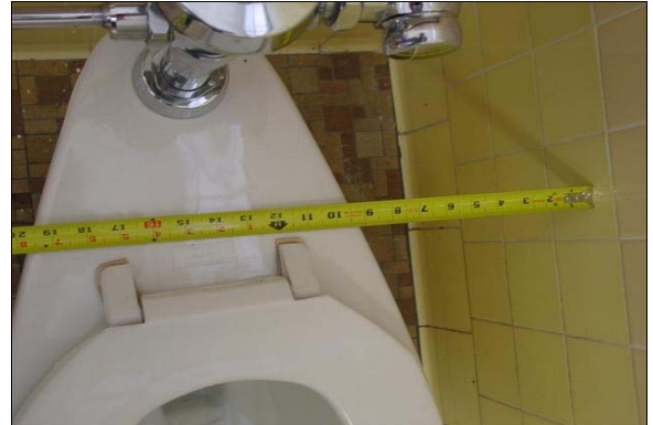
Girls Restroom Building A
