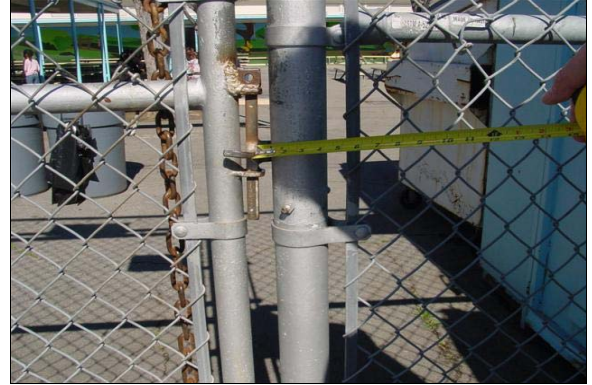
Gate Next to Cafeteria
