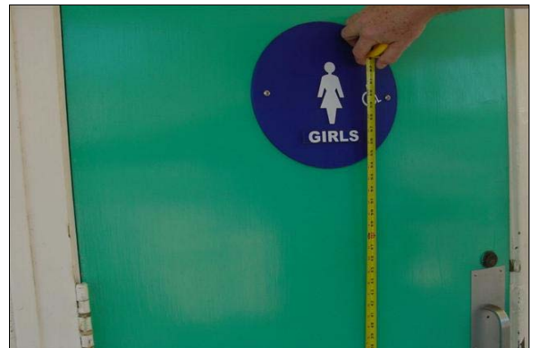
Girls Restroom Building A
