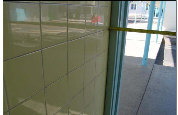
Girls Restroom Building A
