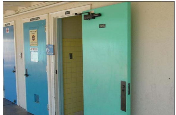
Boys Restroom Building A
