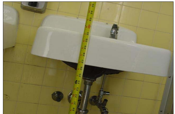
Girls Restroom Building A
