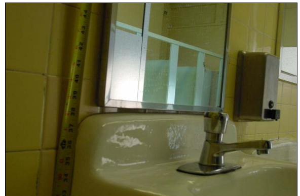
Girls Restroom Building A
