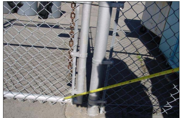
Gate Next to Cafeteria
