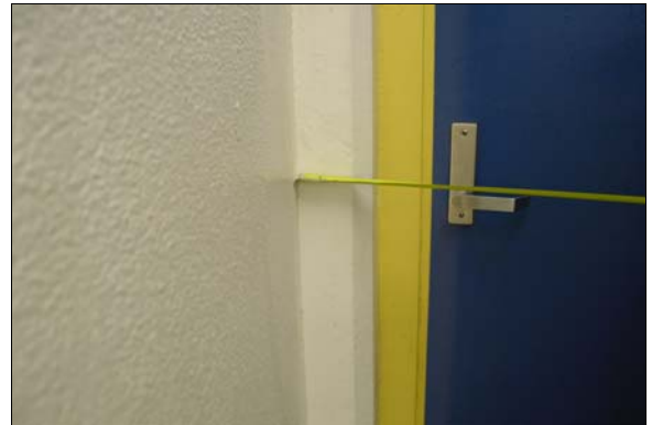
Boys Restroom next to the Small Gym
