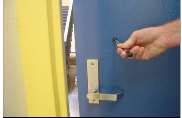
Boys Restroom next to the Small Gym
