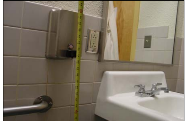
Staff Womens Restroom in the Main Office
