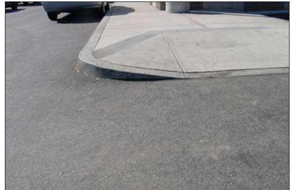
Curb Ramp at the Florence Avenue Parking Lot
