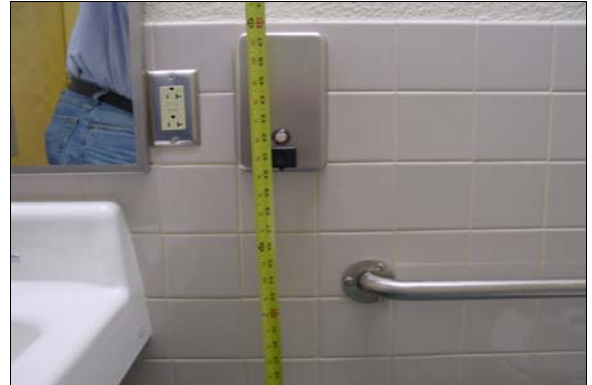
Staff Mens Restroom in the Main Office
