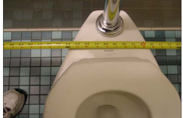
Girls Restroom Across from Room 114
