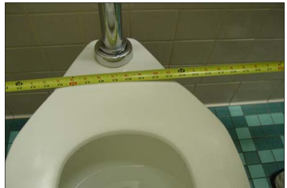
Staff Womens Restroom in the Main Office
