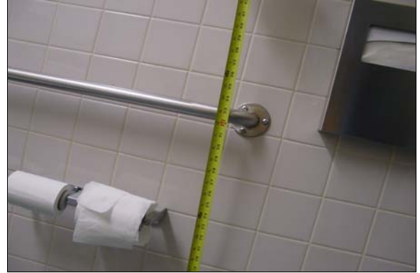
Staff Mens Restroom in the Main Office
