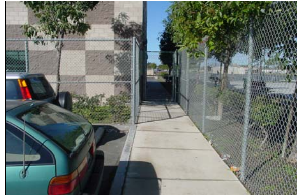
Gate from Florence Avenue Parking to School
