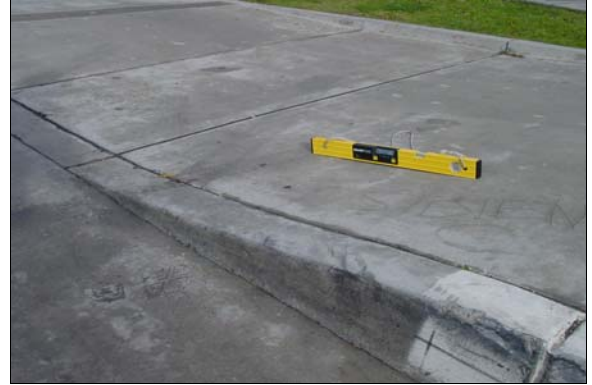
Curb Ramp at the Bus Loading Zone
