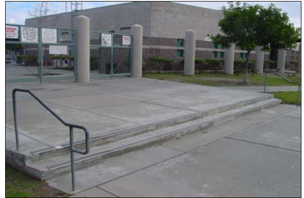
Exterior Stairs next to the Bus Loading Zone
