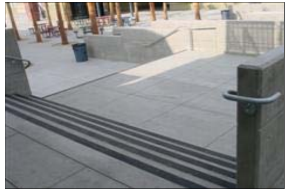
Stairs at Building 3
