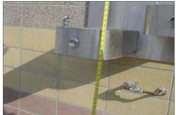
Drinking Fountain Outside Field House Restrooms
