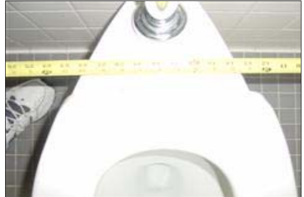
Mens Restroom at Rear of Stage
