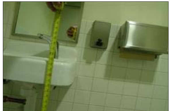
Mens Restroom at Rear of Stage
