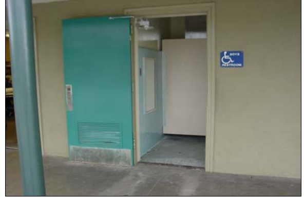
Boys Restroom in Building D
