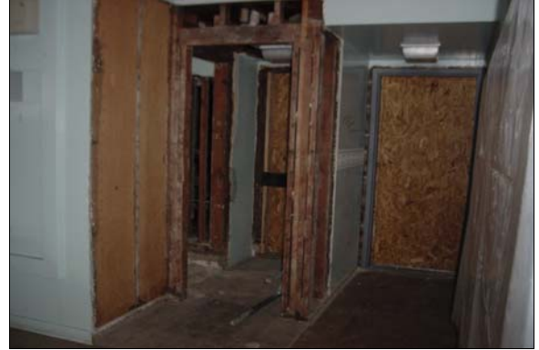
Boys and Girls Restrooms in Building A
