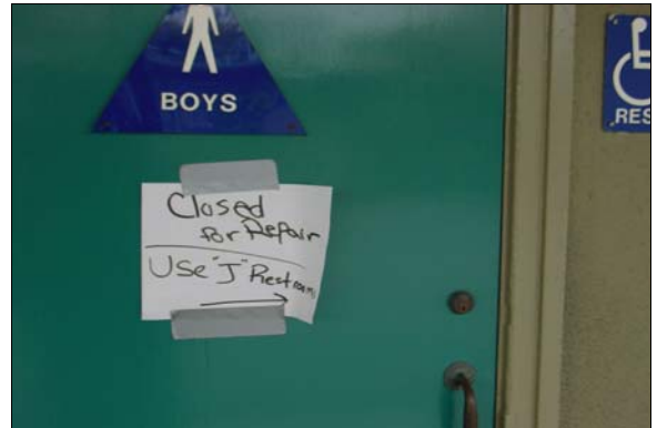
Boys Restroom in Building D
