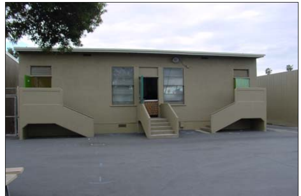
Building J Restrooms
