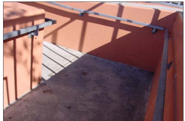
Exterior Ramp at the Main Entrance
