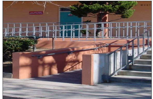
Exterior Ramp at the Main Entrance
